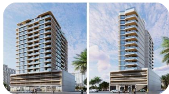
Project: HH034 – Al Jadaf, Dubai - UAE Enterprises LLC Consultant: Future Art Engineering Co. Year: 2025 Scope of Work: Metal Work
