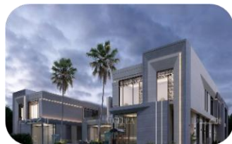
Project: HH027 – District 1, Dubai Consultant: Designer East Year: 2025 Scope of Work: Metal Work
